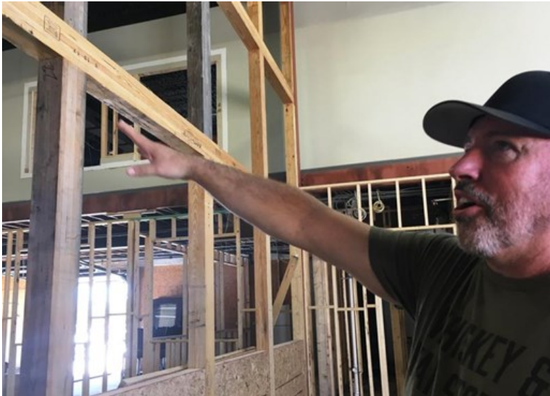
Former Green Beret Scott Neil points to the framework for the glass wall that will separate the American Freedom Distillery from the restaurant under construction.
