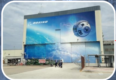
Comm. Crew & Cargo Processing Facility $20M
