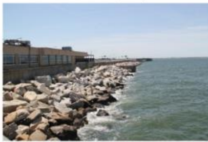
Sea Wall and Riprap
