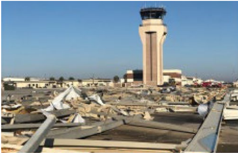
Debris on the Flightline near the Air Traffic Control Tower
