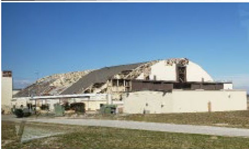
Damage to Hangar 5
