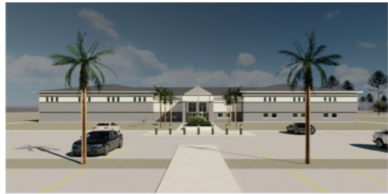
Multi-Unit Armory Gainesville New Construction $21M (100/0)
