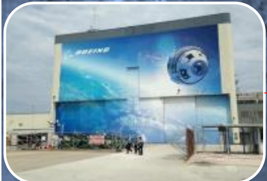
Comm. Crew & Cargo Processing Facility $20M
