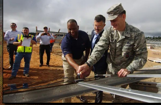
Solar EUL 30 MW output to grid
