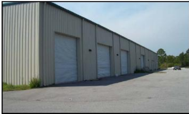
View of East Side of Subject Building
