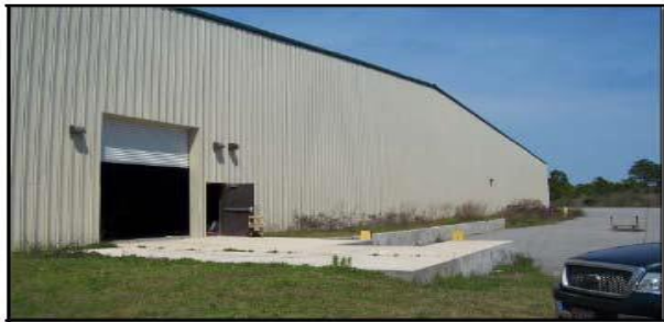
View of South Side of Subject Building
